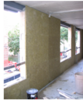
1" Mineral Wool (picture taken prior to steel stud installation)
