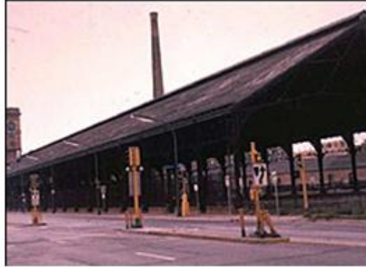
Instead of demolishing the former train shed, it was converted into an indoor ice arena. Photo of indoor ice arena: Audrey Tepper) (Courtesy of National Park Service
